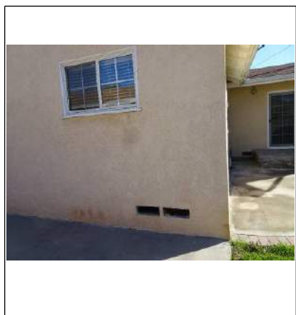
Vent screen missing
