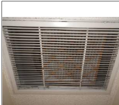
Filter not appropriate size for intake.
